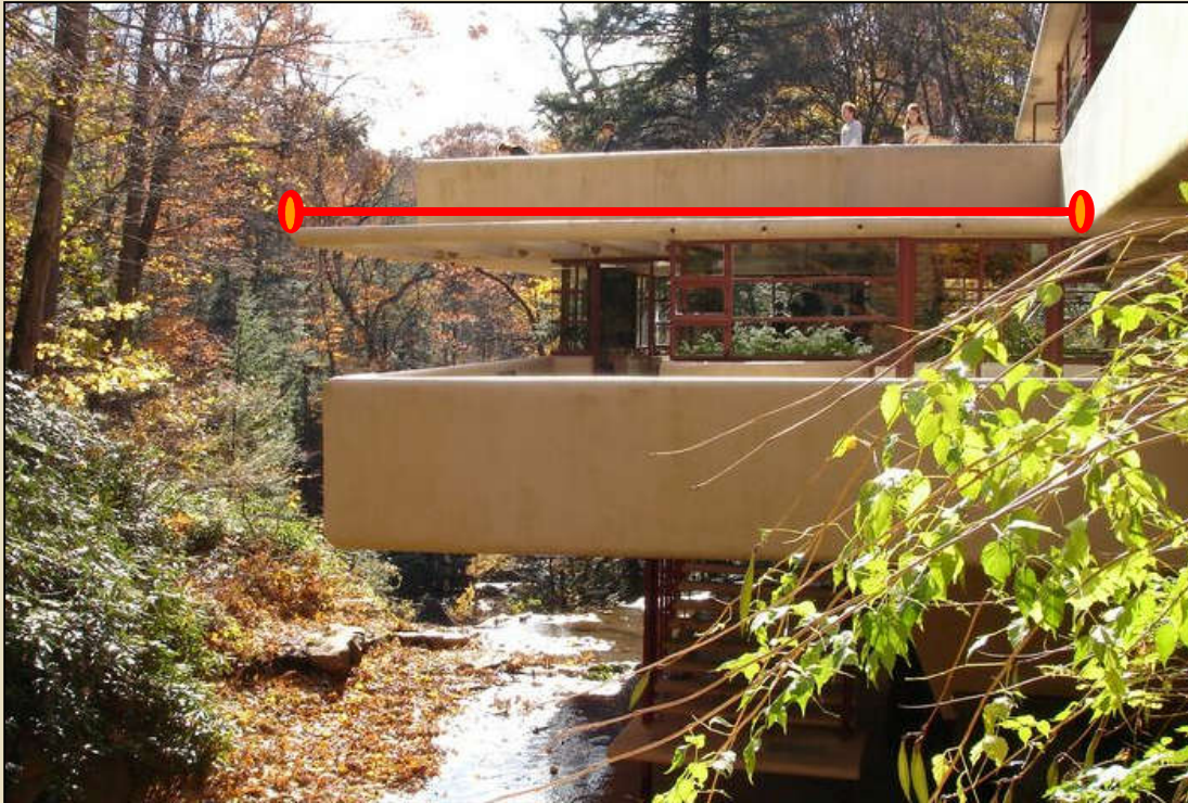
Vila Fallingwater, Pennsylvania, USA, autor. Frank L. Wright; foto: Ing. Cyril Fisher, Ph.D.
