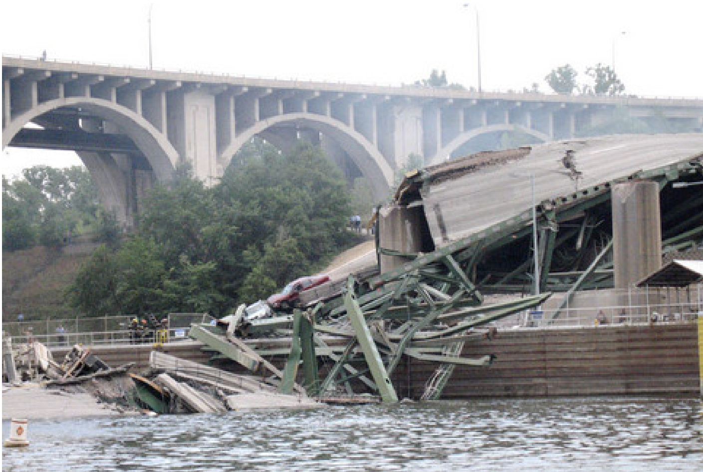
Ruined bridge over the Mississippi, Minneapolis, August 2007
