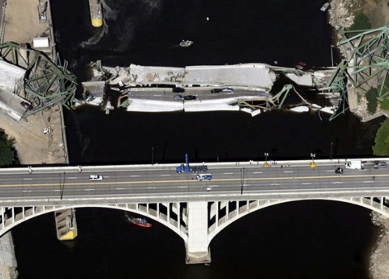
Ruined bridge over the Mississippi, Minneapolis, August 2007
