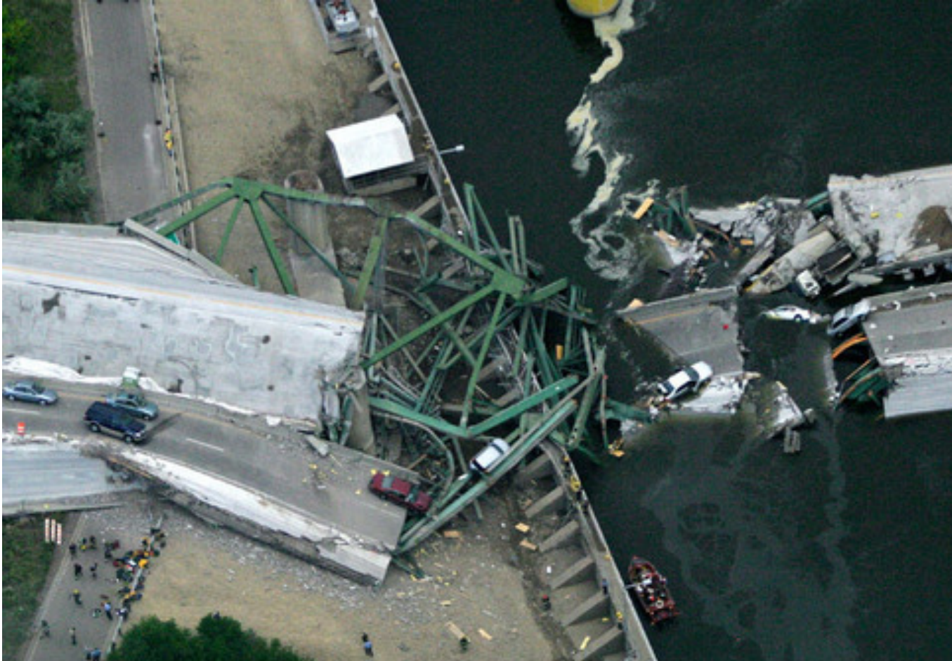
Ruined bridge over the Mississippi, Minneapolis, August 2007
