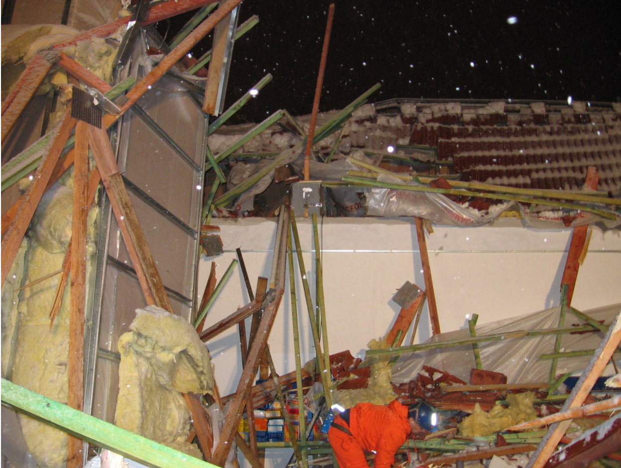
Destruction of a wooden truss in Ostrava, photo: Assoc. Prof. Karel Kubecka
