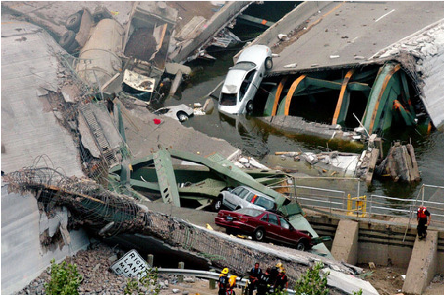
Ruined bridge over the Mississippi, Minneapolis, August 2007
